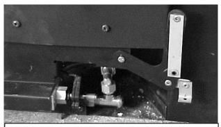
Cut a cross slit in the rubber grommet and feed the appliance onto the 8mm-gas supply pipe. Position the restrictor elbow supplied and mark supply pipe at its cut off length. Remove appliance, cut pipe to correct length, refit appliance and make gas connection with restrictor elbow use 15mm A/F spanner taking care not to apply any force to the gas control spindle as above. Ensure the restrictor valve is opened and its cap replaced tightly.
