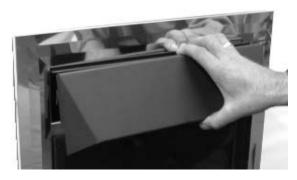
Fit the convector hood to the firebox by engaging the two mounting hooks into the relevant slots in the firebox. The hood should be pressed inwards and downwards to secure into position.
