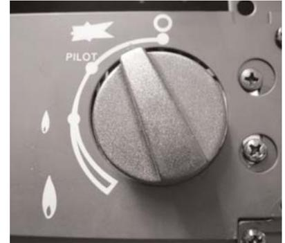
A safety interlock prevents re-ignition of the pilot flame until the thermocouple has cooled sufficiently to allow the magnetic valve unit to reset itself.
